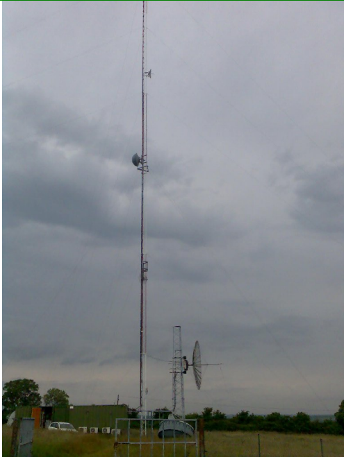
Transmitter Site Photo
